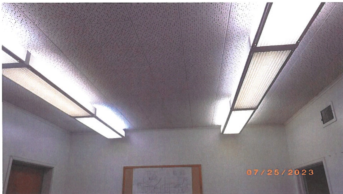
Photo 12: Typical suspended acoustical ceiling. (Reclamation/C. Patane)
